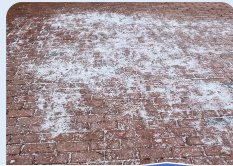
Over applied road salt on a walkway
